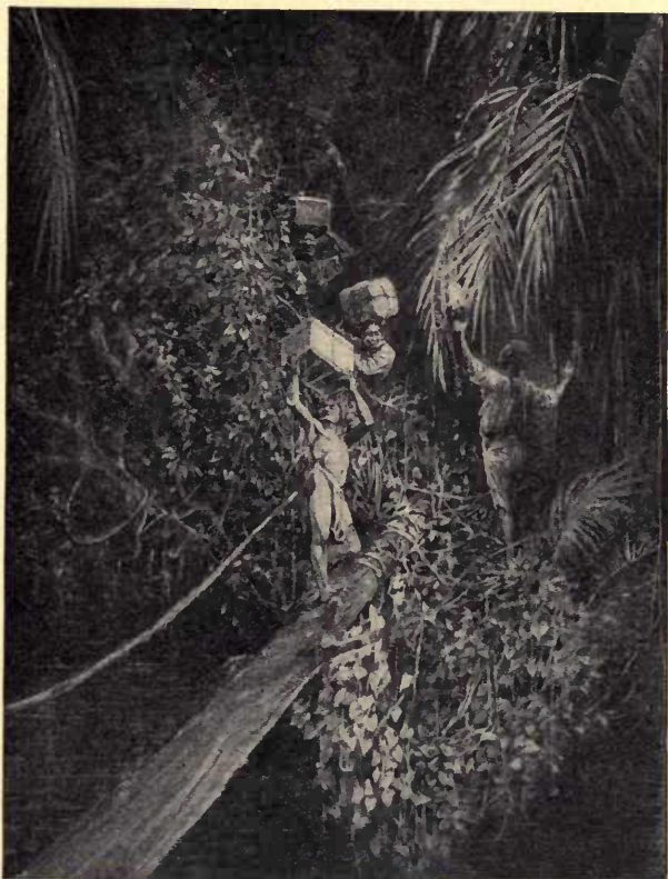
An Improvised Bridge.
